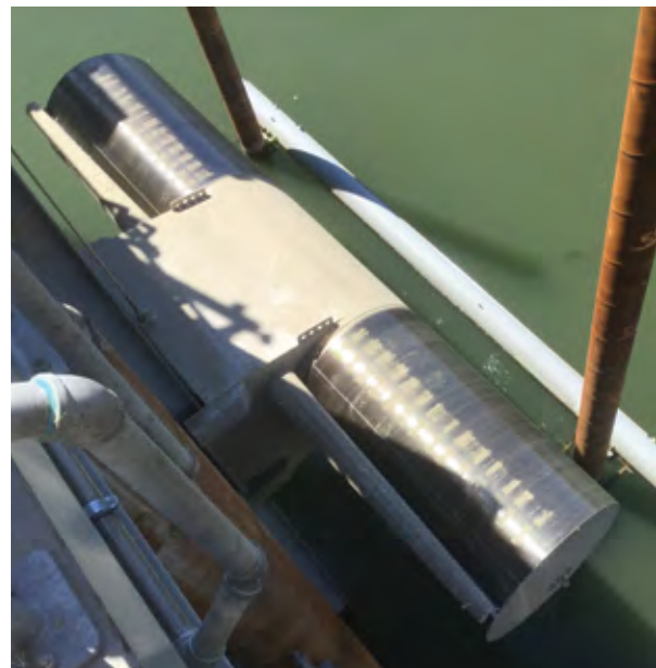
A self cleaning rotating pump screen is one of many different types of screening solutions available to keep debris and fish in the river.
