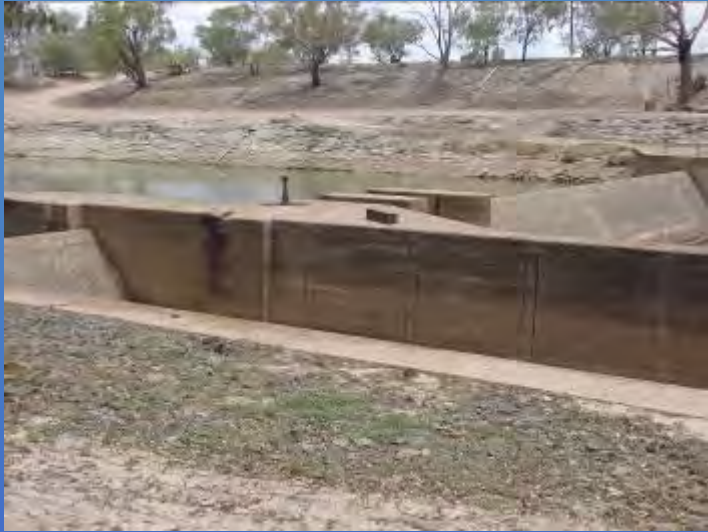
Lock and weir at Bourke
