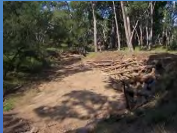
After - Shawns Creek log bank revetment
