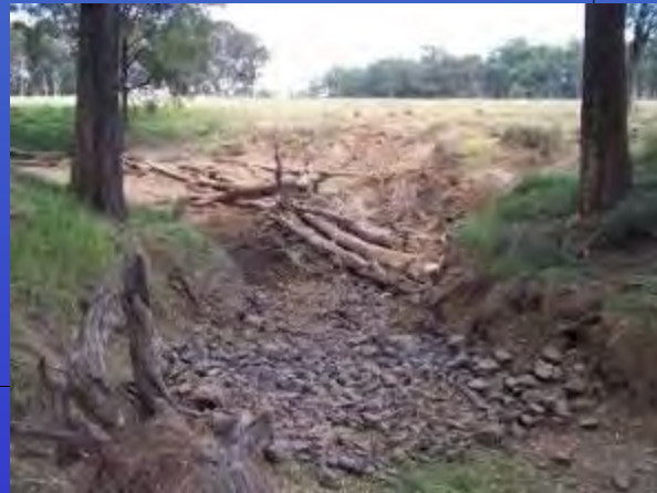
After - Shawns Creek - rock shute and bank revetment
