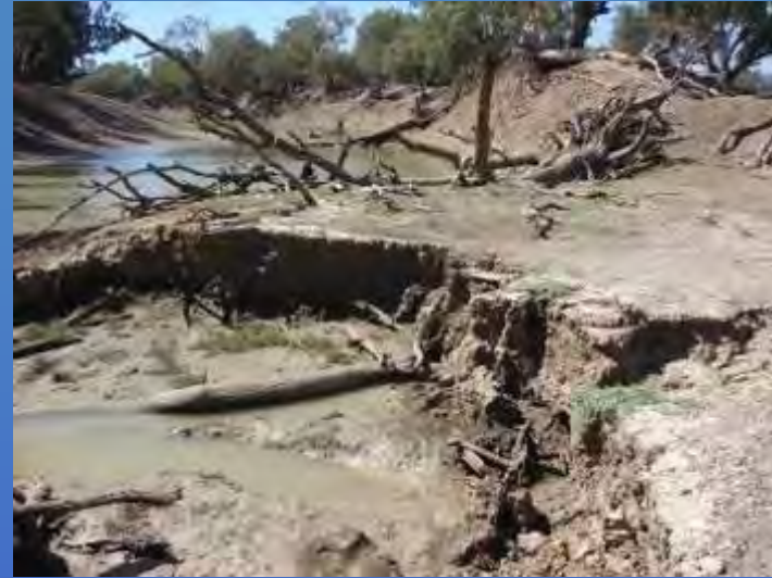
Bank failure – Barwon River
